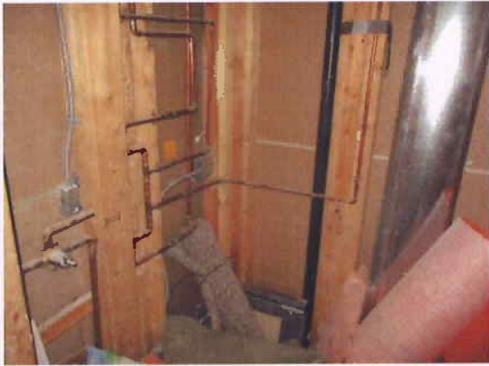
Roughed in plumbing and studs for a shower
