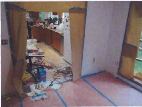
Construction in progress?
