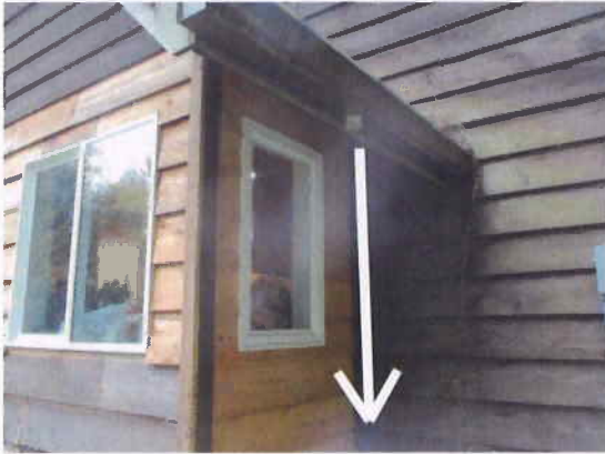
Missing downspout
