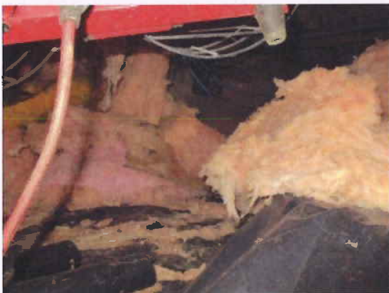
Pulled down insulation
